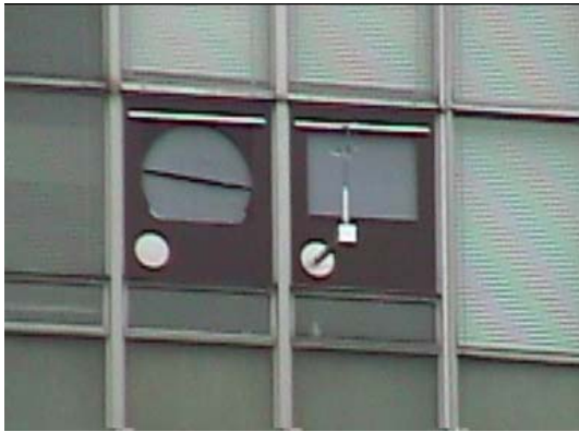
Figure 6: Driving-rain gauges in the west facade of the Main Building at position P5 (left, d.r. gauge II with wiper) and P4 (right, d.r. gauge I without wiper).
